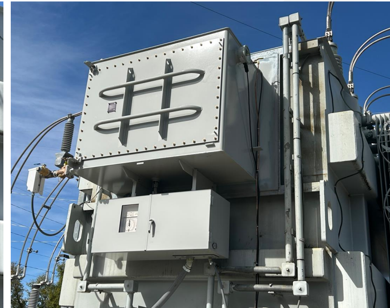
After LTC Replacement
