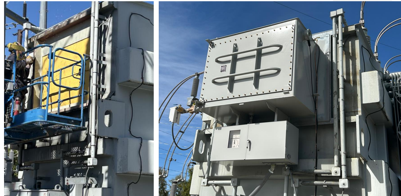
After LTC Replacement
